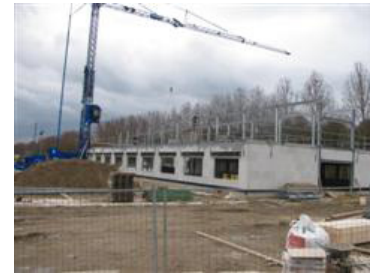
Construction in progress
