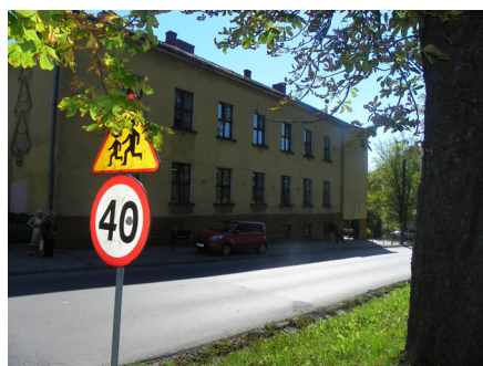
Primary school building in Jordanów
