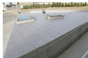
Triangular fuel silo
