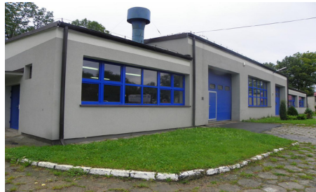
Technical workshops building
